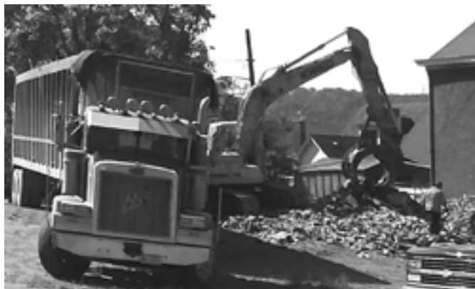
A house being demolished in a Pittsburgh neighborhood
